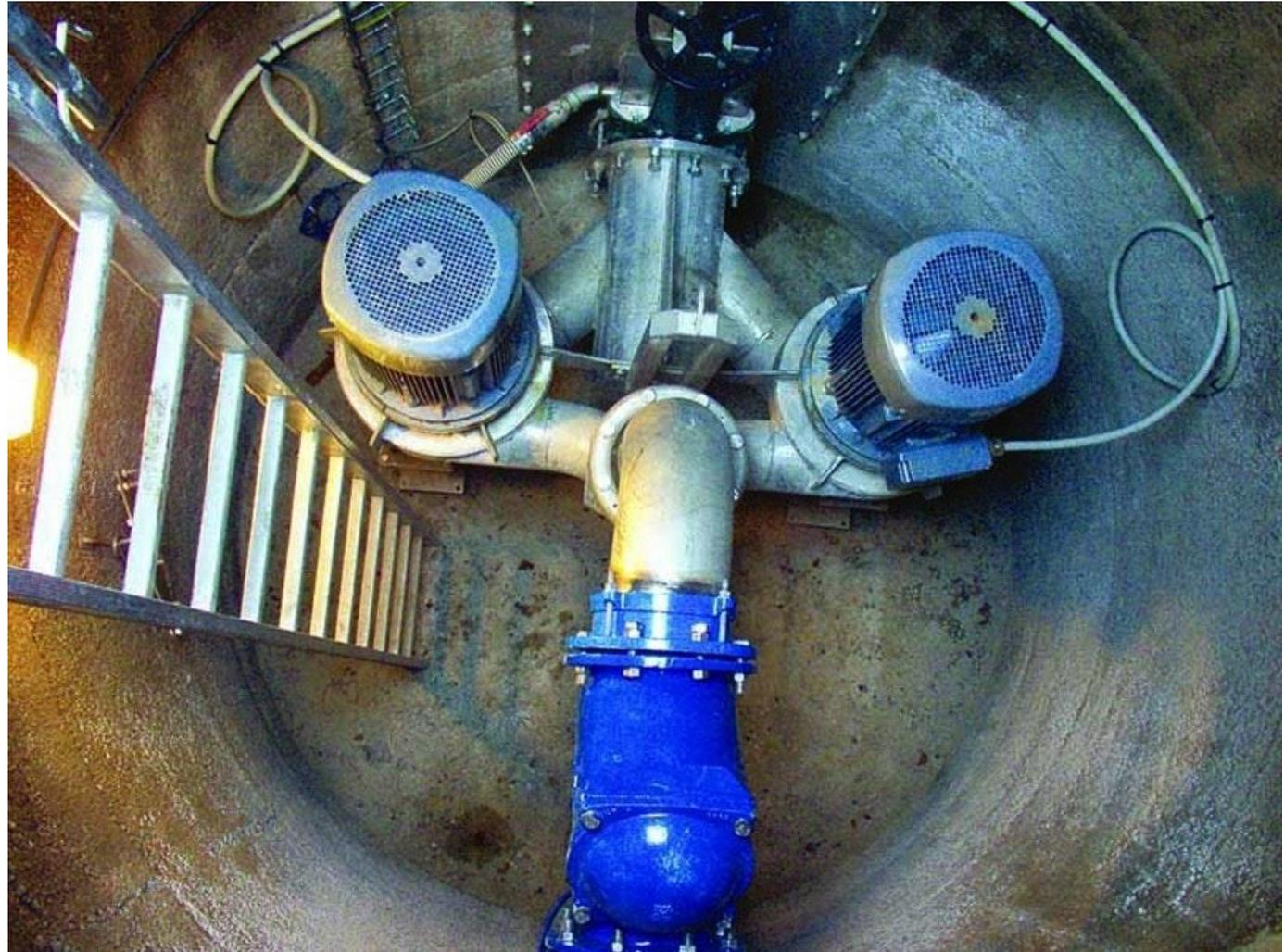
Wet well showing submersible pump lifting/lowering, and floats.
