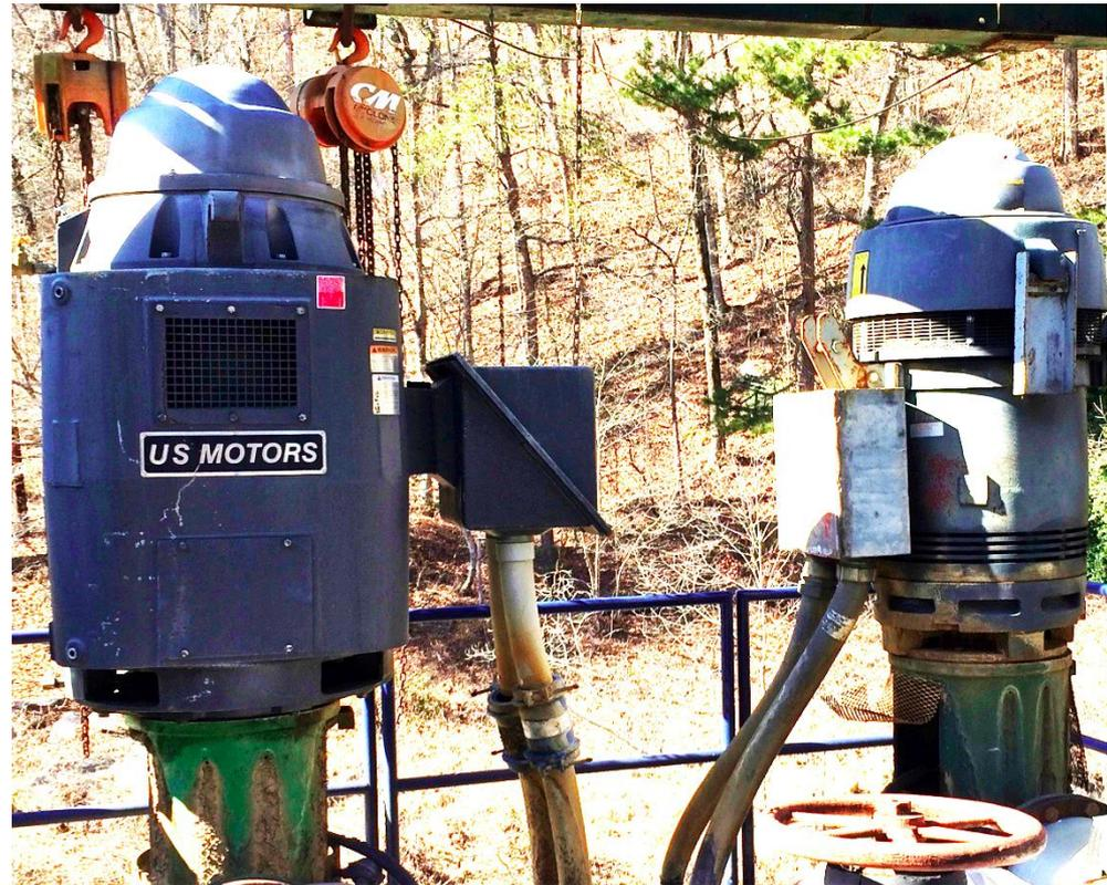
Raw Water Pumps are usually sized for the maximum capacity of the Water Treatment Plant. Rarely is this much horsepower necessary. This are a very good candidate for VFDs.
