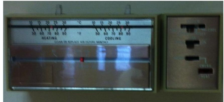
If these exist in your facility, it is time for an upgrade! Installing programmable thermostats can reduce the HVAC energy usage by 50% or more. It is rare to see any programmable thermostats in a water or wastewater facility. This is an easy fix.
