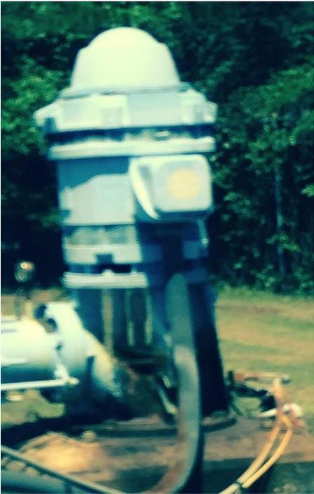
Let us assume this vertical turbine 40 Hp 89.5% efficient motor fails. We have to make a decision on whether to get it rewound, replace it with standard efficiency, or replace it with high efficiency.
