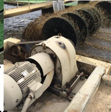
**These systems, called oxidation ditches (street name “orbitals” or “racetrack”) use a rotating disk or brush mechanism that provides aeration and velocity. These are inefficient and very maintenance intensive. An efficient upgrade would separate the aeration from the velocity component.**
