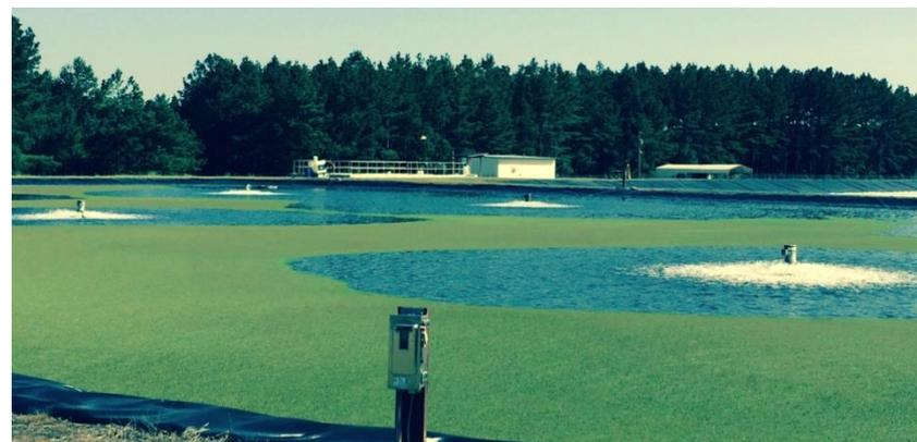
**For lagoon applications, floating aerators are popular, but they are horribly inefficient. Most have no feedback loop so they run 24/7 or are on timers that are based on worst case scenarios (a one time anomaly causes too defensive operation) .**
