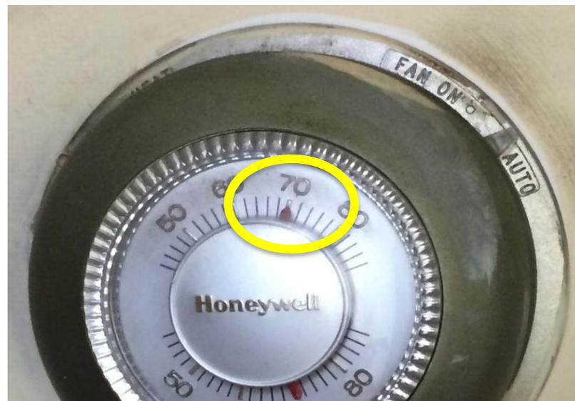
It is bad enough that these are manual thermostats and run continuously, but the set points are also low. At 2% - 5% power use for every degree, the 65F set point is increasing consumption 16% to 40%.
