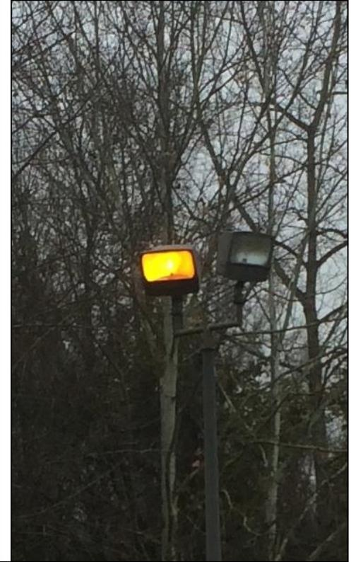
**3 out of 4 outdoor HPS area flood lights were stuck on. This is usually indicative of a faulty or dirty photo eye. These are good candidates for an LED upgrade.**
