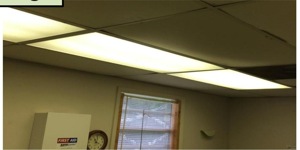
This lighting is the older magnetic ballast T12 lighting, which is inefficient, can cause headaches and is becoming obsolete.
