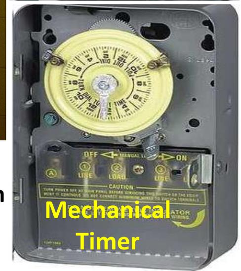
Electrical Resistance Water Heaters should only be scheduled during normal work schedules. The mechanical timer has been commonly used for water heaters for many years, but the electronic timer does not lose the timer settings on a power outage and can have battery back-up. Natural Gas should be considered if possible.
