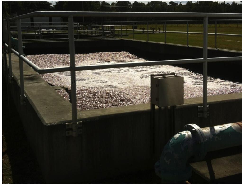
The blowers for the aeration of this “activated sludge” plant run 24/7 no matter what the load on the plant is. This would be a good opportunity for VFD control based on the actual DO level. Some control systems can look at the influent and anticipate what the load will be and set the DO accordingly. Excess DO is excess energy use!
