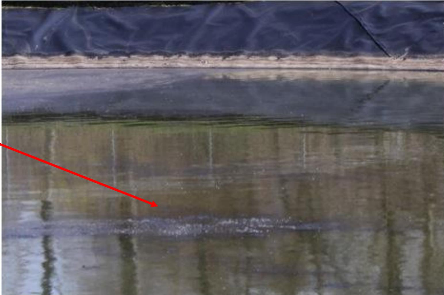
Bubbles due to gases released from anaerobic decomposition of sludge.
